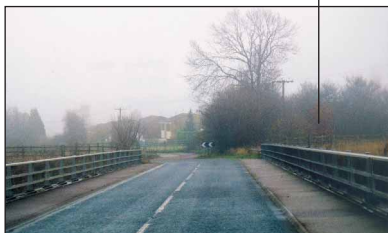
View looking east from A417 bridge towards Featherbed Lane - access to site to right of bridge
