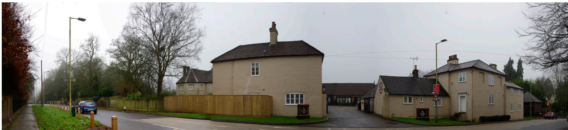
Panoramic view from north-eastern boundary facing south
