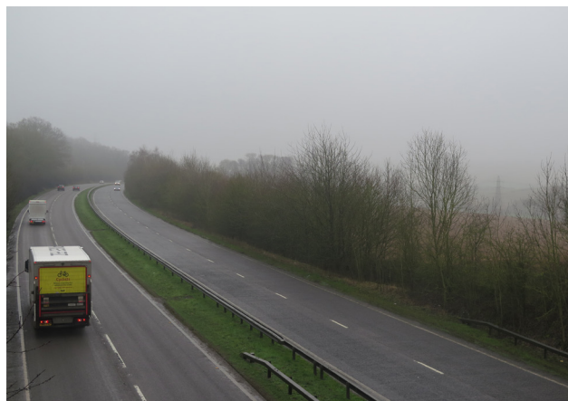
View of southern boundary planting adjacent to the A41
