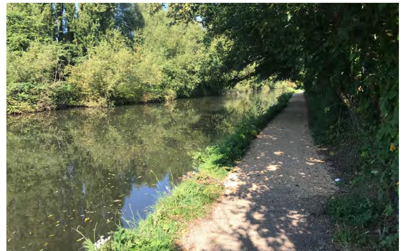
Figure 10 Resurfacing improvements to the Grand Union Canal (June 2023)
