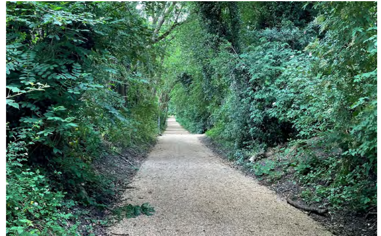
Figure 9 Phase 2 Resurfacing on the Nickey Line (2023)
