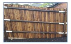
When we erect a new fence along the boundary between a garden and a public footpath it will usually be approximately 1.8 metres (six feet) high and constructed of feather-edged wooden boards.
