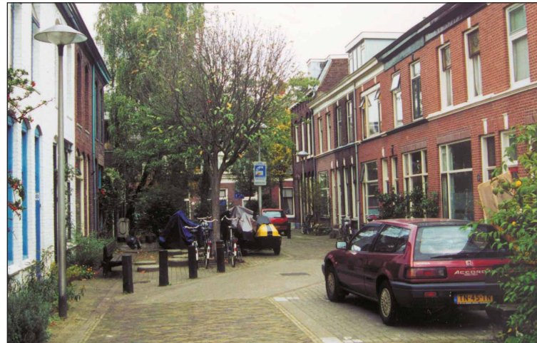
Shared surface or ‘home zone’ streets create safe and attractive environment (Dutch example)
