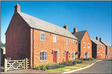
New development should aim to create a well defined frontage and variety to the roofscape of the street
