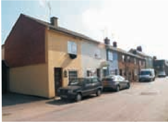
Cottages on the east side of Trooper Road
