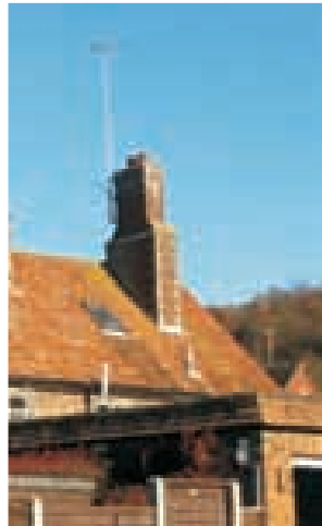
Rooflights visibly interfere with roofscapes
