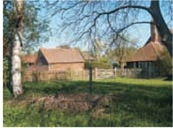
Simple tiled roofs to barn and outbuilding, Stocks Road
