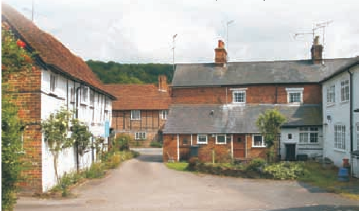
Courtyard to rear of the Greyhound Cottages
