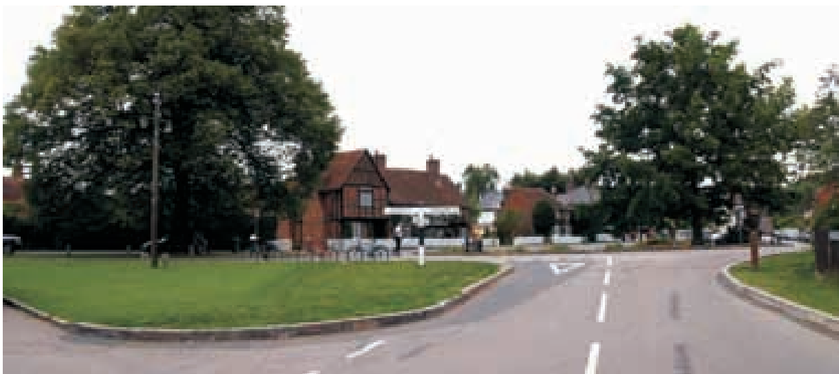
This photograph shows the loss of the lane to the left of the signpost. Some of the unobtrusive kerbing around the Green has also now unfortunately been raised.
