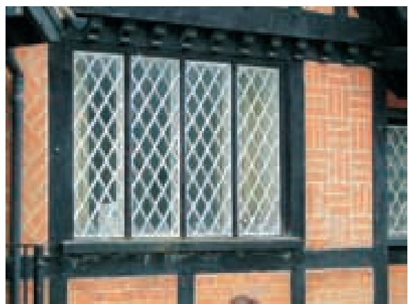
Cast iron diamond lattice paned windows
