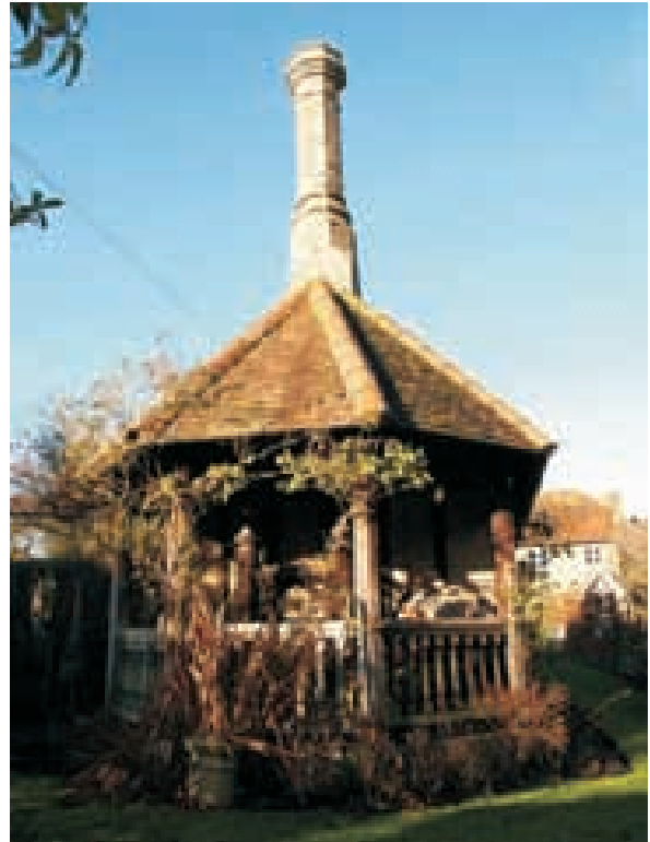
Mid C19th Well house and communal bakehouse, listed Grade II
