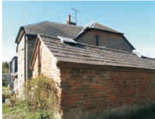
Large slates used on outbuilding, Barrack Row
