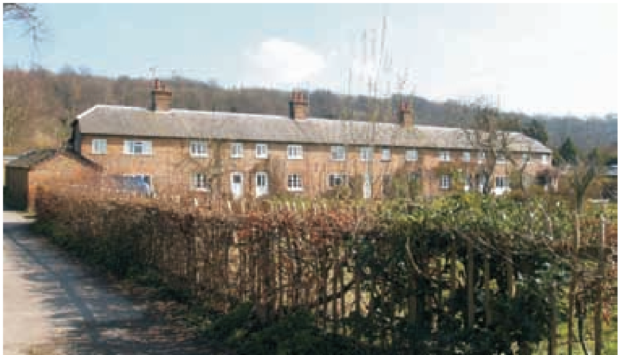
Barrack Row, an example of locally listed buildings
