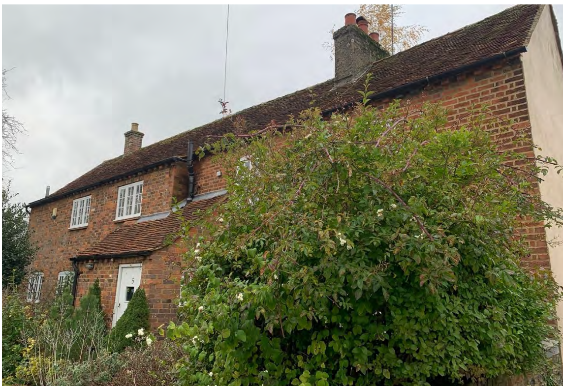
Figure 7: No 5 Church Street, Mid C19 th , later extended brick cottage
