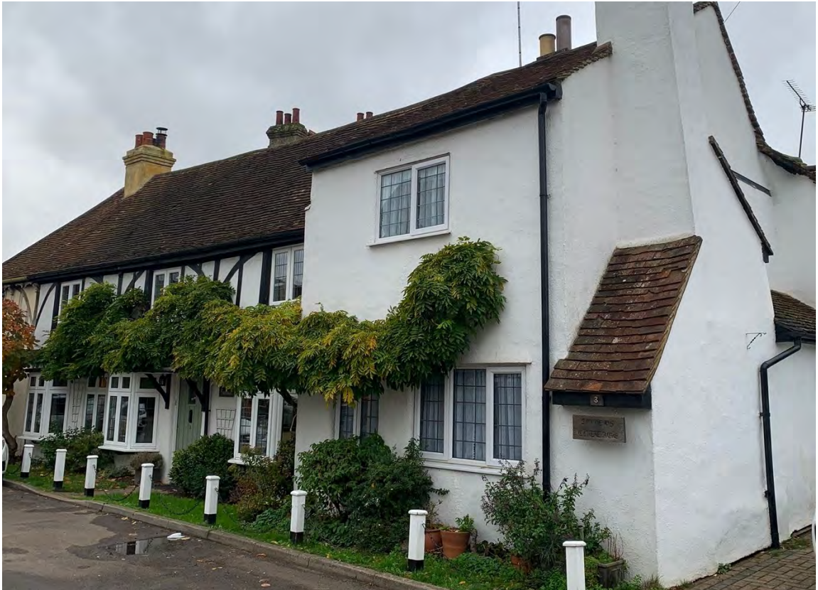
Figure 9: Tiled roof dominates in conservation area
