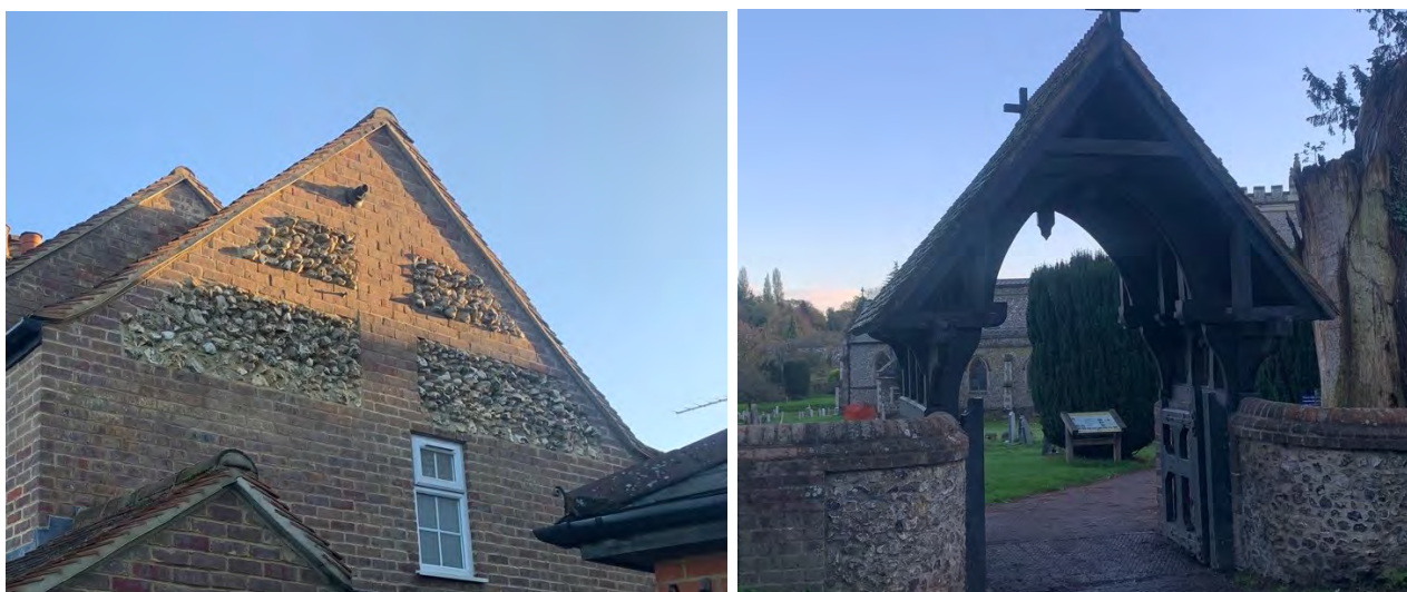
Figure 8: Flint used in modern gable wall (left) and St Lawrence church yard wall (right)
