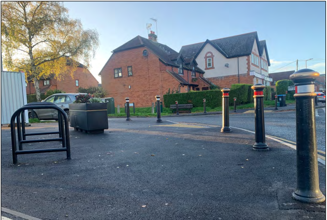
Figure 48: Cycle stands in High Street, and dropped kerbs with tactile paving
