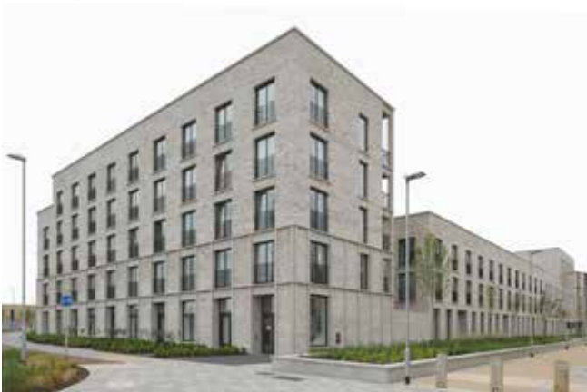
Ryle Yard, NW Cambridge. Maccreanor Lavington. Photo: David Grandorge
