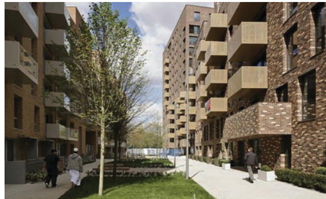
St Andrews, Bromley by Bow. Maccreanor Lavington. Photo: Tim Crocker
